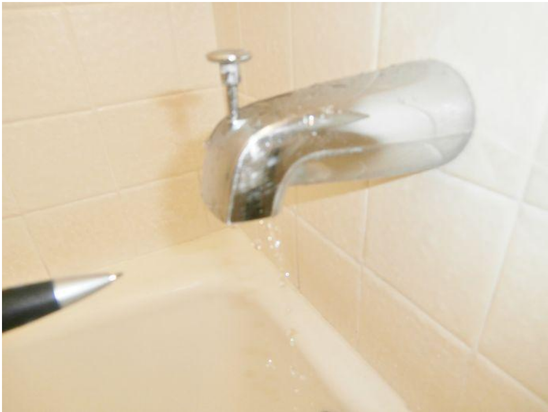
Bathroom #2 Hall downstairs / Shower/Diverter leaked
