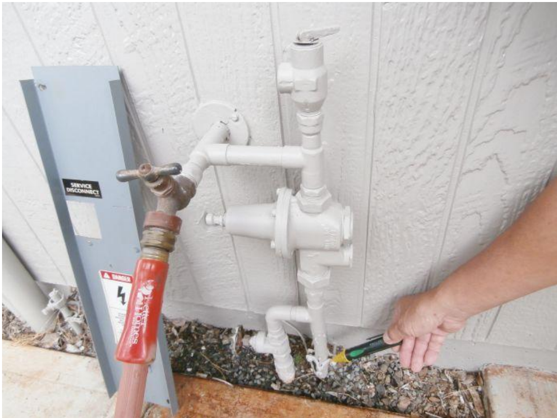
Plumbing / Water pressure valve
