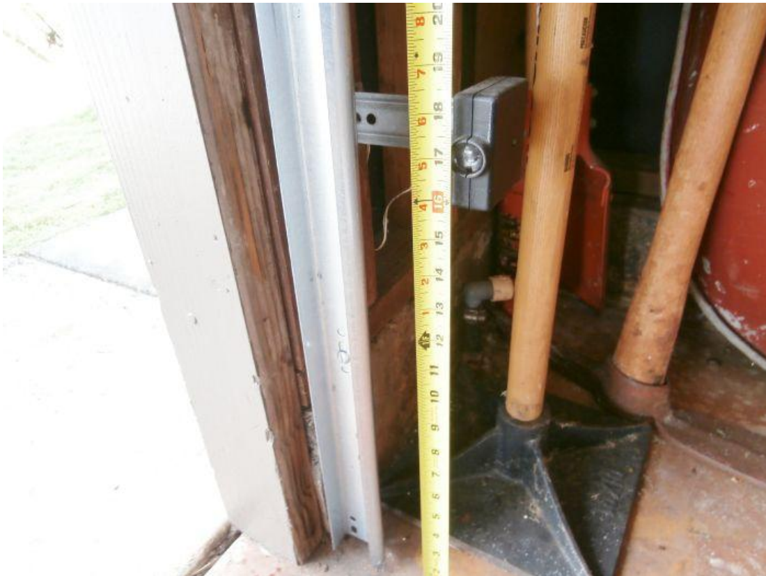
Garage / Infrared Sensors
