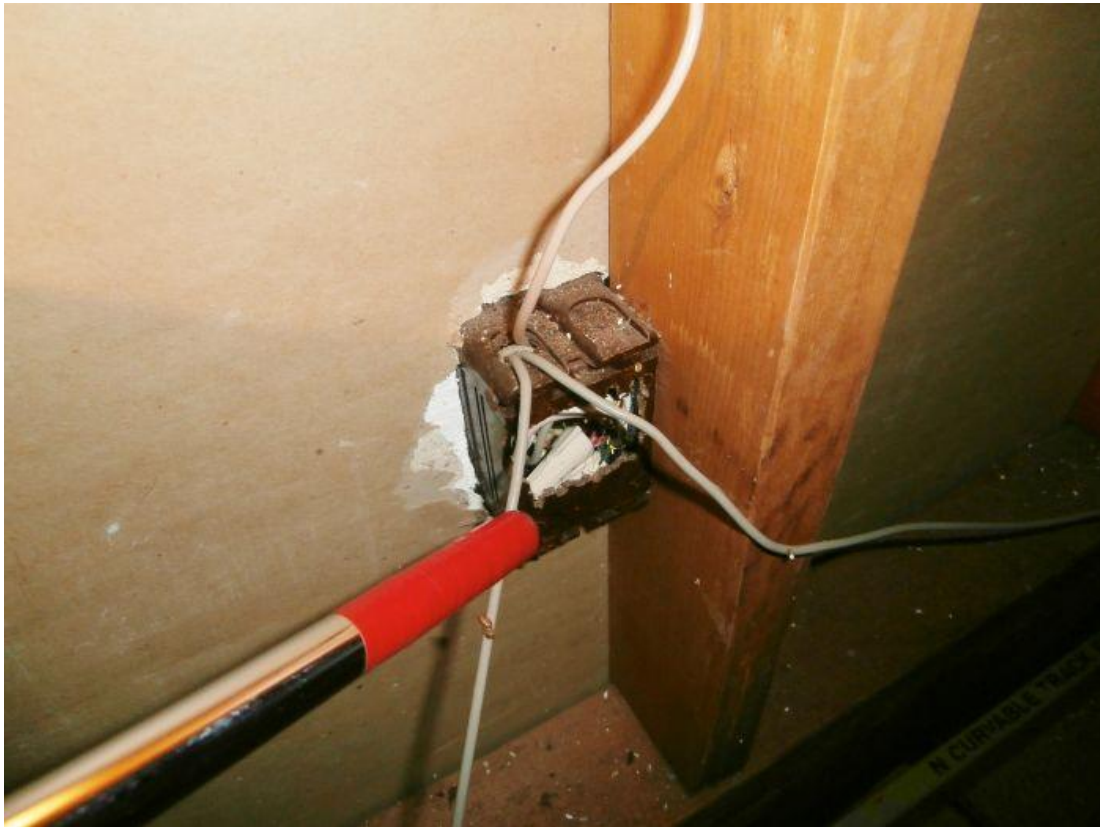
Attic / Damaged cable junction box.
