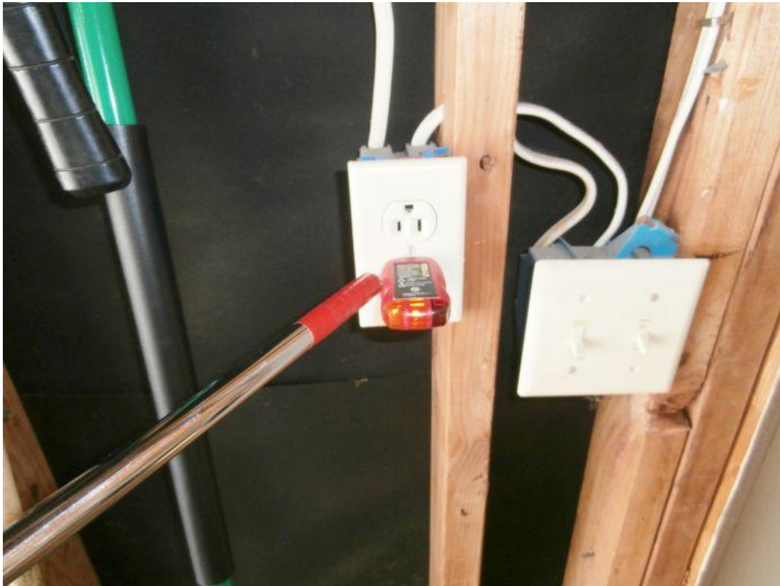
Garage / Garage Electrical hot/neutral reverse
