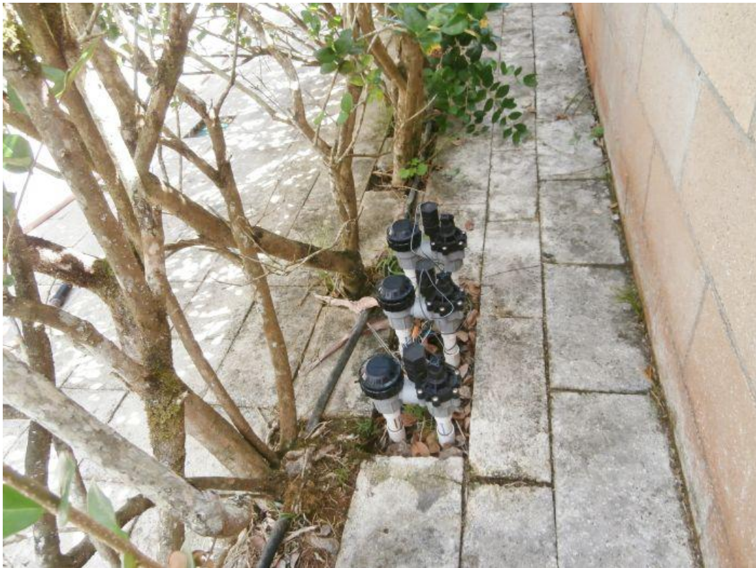
Grounds / Lawn sprinkler/anti siphon valves
