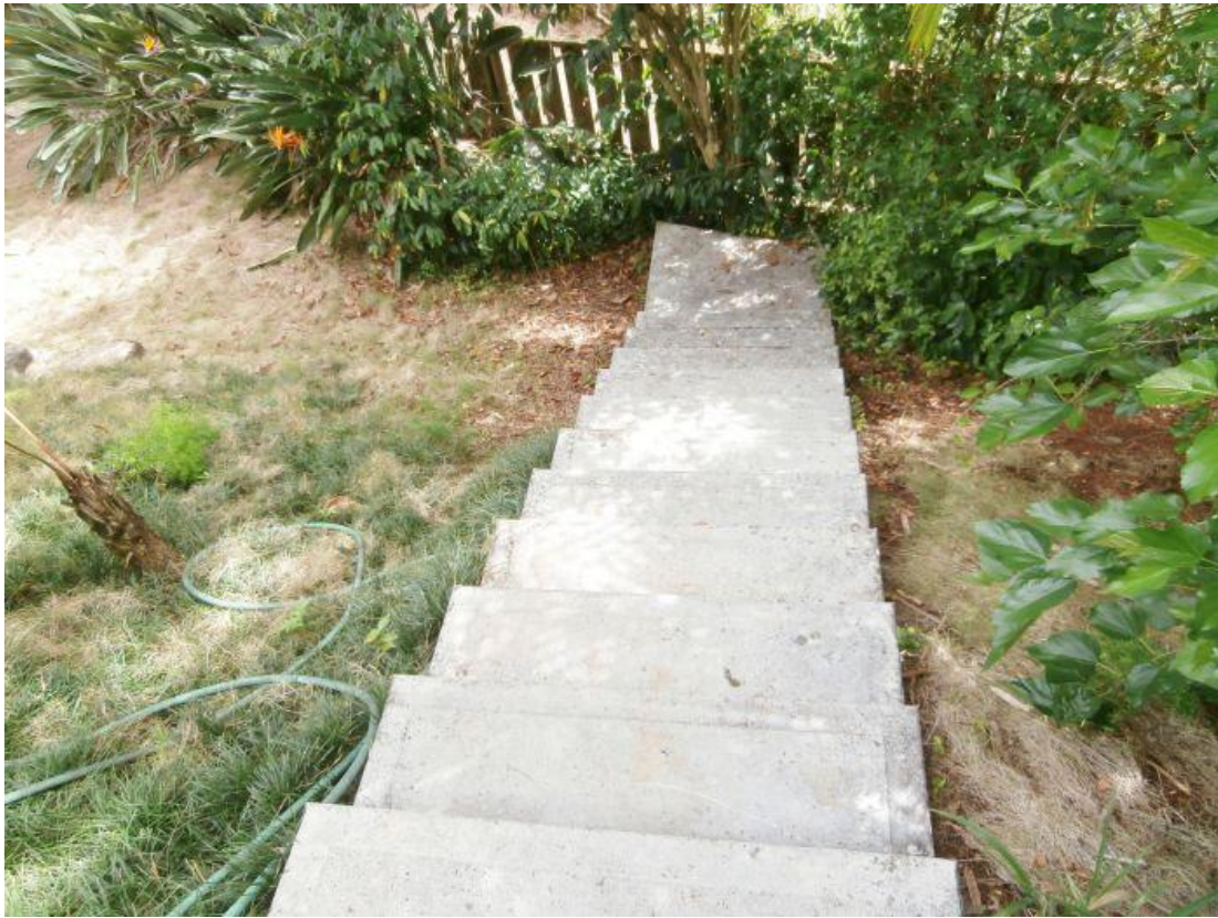
Grounds / Exterior Stairs missing hand rails
