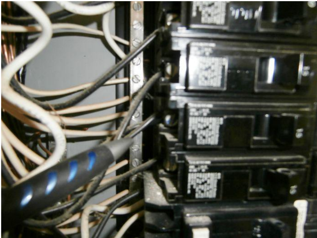
Electrical / Sub-panel breaker double-lugged.
